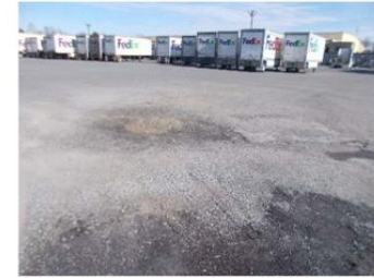
Photo #2 Exposed subgrade in high severity pothole observed at loading area entrance.
