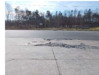
Photo #3 High severity scaling with chunks of concrete being dislodged from the concrete apron at loading area entrance off of CSX Way.
