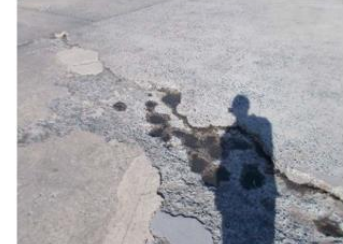
Photo #2 Exposed subgrade in high severity pothole observed at loading area entrance.
