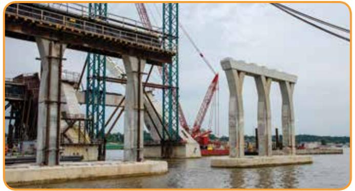
Temperature sensors are connected to the yellow remote radios (tied to the scaffolding in the upper left of the photo) that sends readings to the team.
