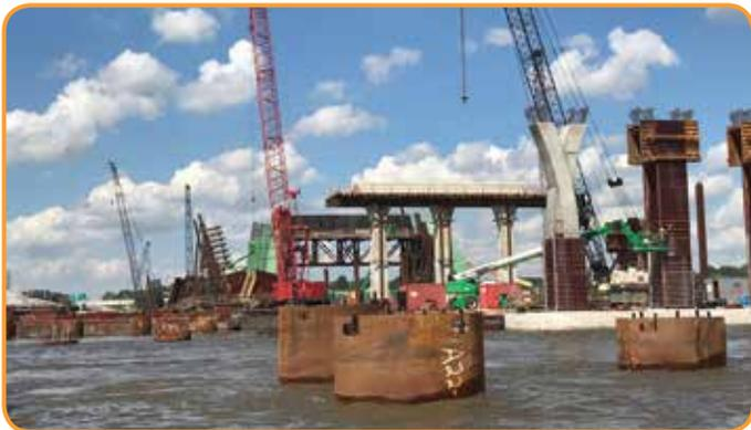
Various stages of construction for the concrete substructures and foundations for the I-74 bridge project, including deep foundations, footings, columns, and pier caps. In the background are the substructures for the new bridge arches.
