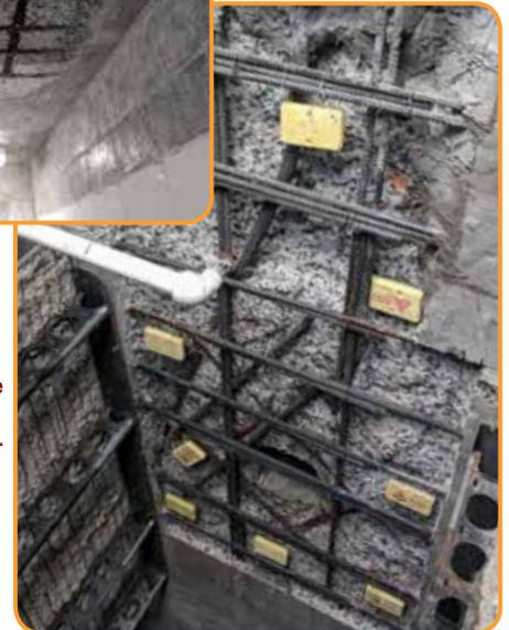
the steel corrodes, allowing for extended service life of the steel. Observations were performed to check the connection between the sacrificial anodes and the steel, the cleaning and coating of the steel reinforcement, and the installation of the mortar to confirm the repair mortar was well bonded to the substrate.
