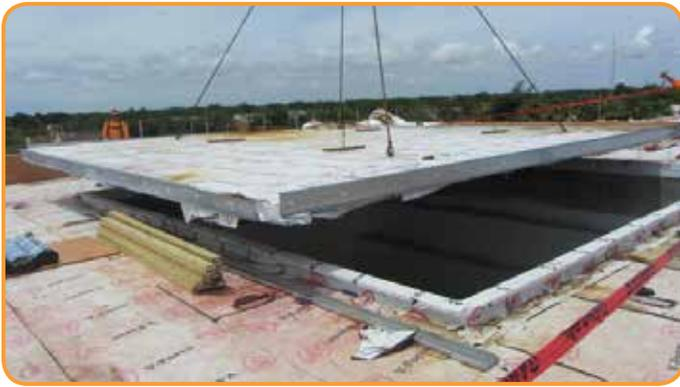
**The cover for a proton therapy chamber is lowered into the building through the roof.**
