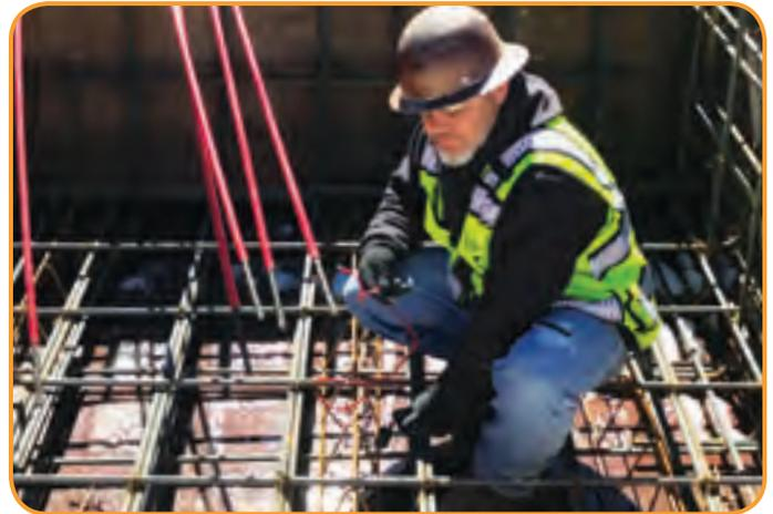
Mike Poore, a construction inspector in our Denver office, installing a maturity meter logger onsite.
