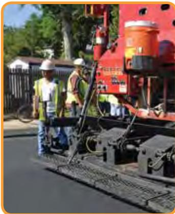
The hot-in-place asphalt surface Recycling Single Pass Method is employed here. The system saves clients time and money by completing HMIPR process in one pass. Photo courtesy of Cutler Repaving.
