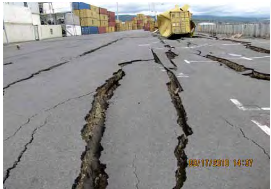
Figure 6. Liquefaction and lateral spreading-induced damage at the Port of Coronel (photo: GEER, 2010).
