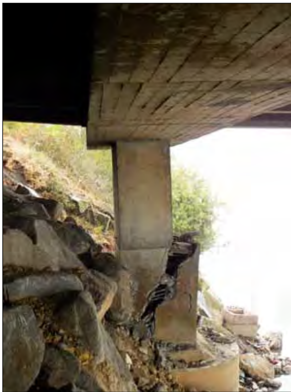
Figure 26. Shear failure in a column in northern approach to Juan Pablo II Bridge across Bio-Bio River, Concepción, due to lateral spreading and the propping action of the superstructure at the top of the column (photo: J. Arias).
