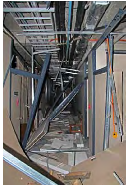
Figure 19. Nonstructural damage in the Talca Supreme Court building constructed in 2003 (photo: E. Miranda).
