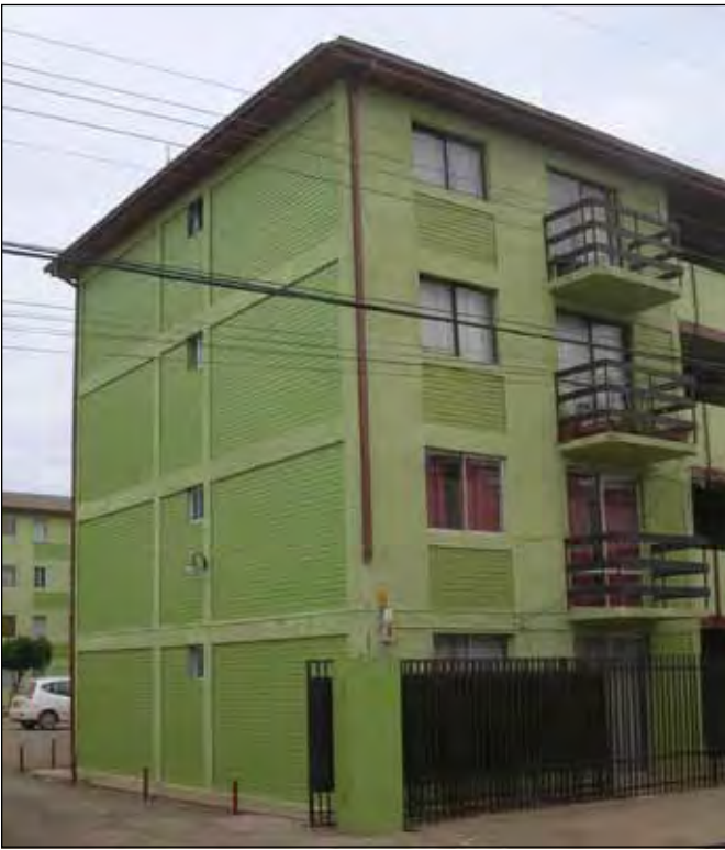
Figure 14. Engineered confined masonry apartment building, showing confining elements at boundaries of walls and openings (photo: M. Astroza).
