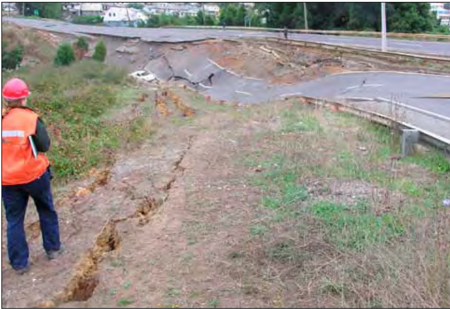
Figure 7. Slope failure on Route 160 in Lota (photo: GEER 2010).
