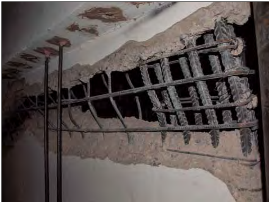
Figure 16. Wall damage, Santiago. Note the 90-degree bends on the transverse reinforcement (photo: J. Wallace).
