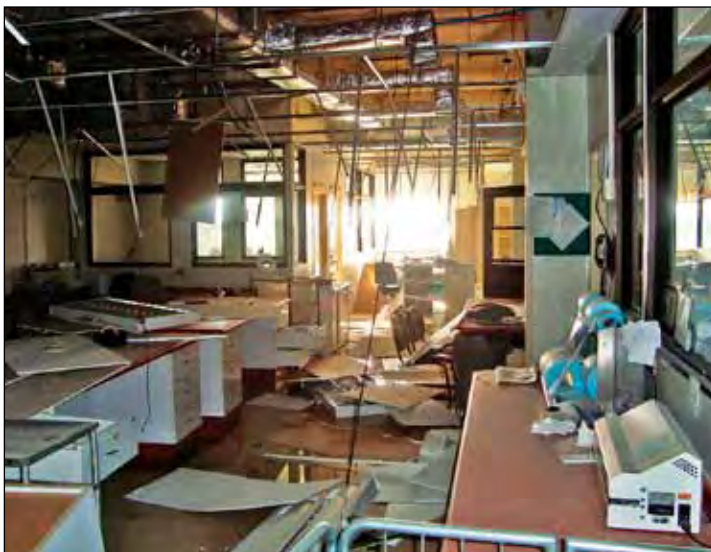
Figure 21. (a) Ceiling collapse and nonstructural damage in Chilean hospital (photo: W. Holmes), and (b) tedious reorganization of medical records three weeks after the earthquake (photo: J. Mitrani-Reiser).
