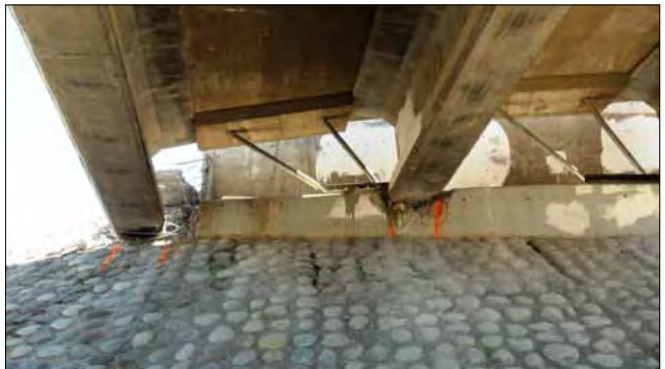
Figure 24. Lateral movement of the superstructure of Las Mercedes Bridge across Route 5 near Rancagua, due to absence of end diaphragms and transverse shear keys. Note extreme deformation of vertical seismic bars and damaged curtain walls (photo: Ministerio de Obras Públicas).
