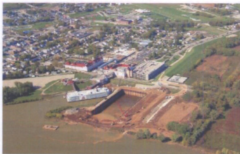
Aerial site photo of the Open Cell sheet pile wall construction (November 2007).
